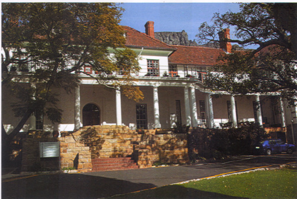
Eco Insulation was successfully used in the upgrade of the insulation system for St. Cyprians school in Cape Town
