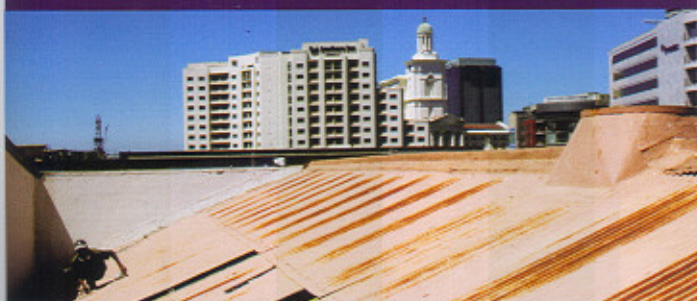
Removing individual roof sheets to allow access into the roofspace
