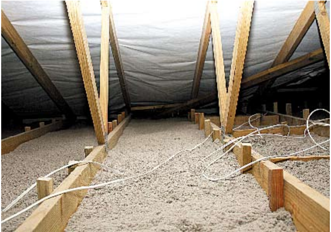
Roof interior - Eco-insulation is easy to install
