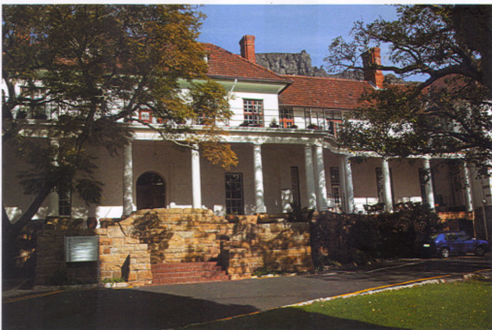
Eco Insulation was successfully used in the upgrade of the insulation system for St. Cyprians school in Cape Town
