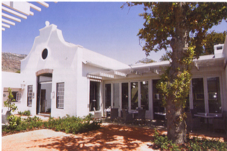
Eco-Insulation was recently used to insulate the extensions to Catharina's Restaurant in the Constantia Vineyards.
